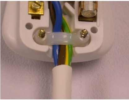
Cable not being gripped.
